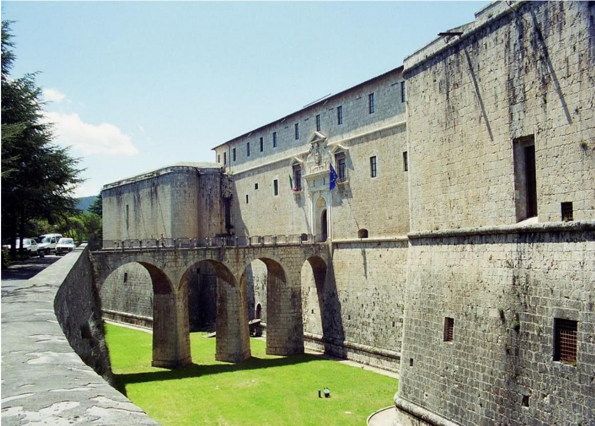
Fig. 4. L'Aquila, Italy: Seismological Observatory is located in the deep basement of this castle.
