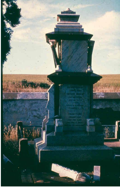
Fot. 4. Contemporary photo of the deformation of the monument; earthquake in Tulbagh-Ceres, South Africa, 29 September 1969 (after R. Teisseyre's Master Lecture).
